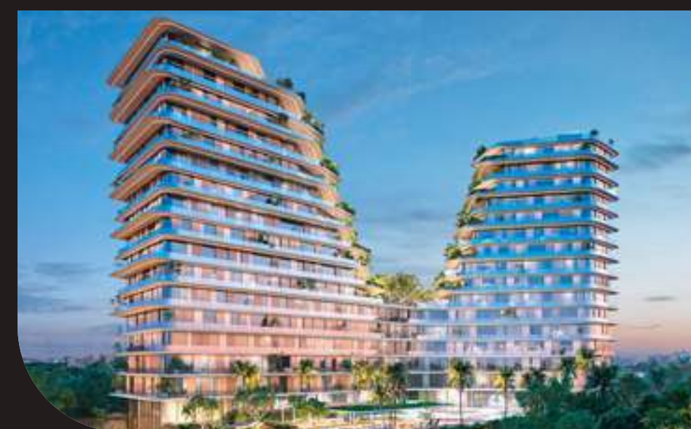
Light Tower / México
