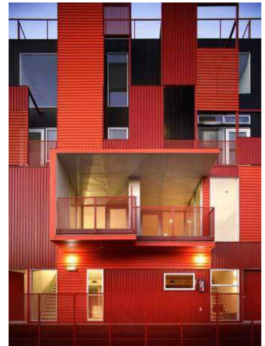
Formosa 1140 / Lorcan O'Herlihy Architects
